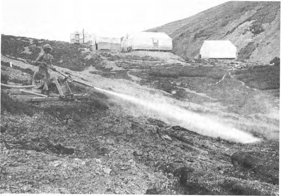
Plate IA. Hydraulicking trenches at the Chappelle property.
