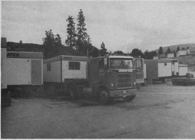
Some of the 27 accommodation units being built at Atco Pacific's Pentiction plant
