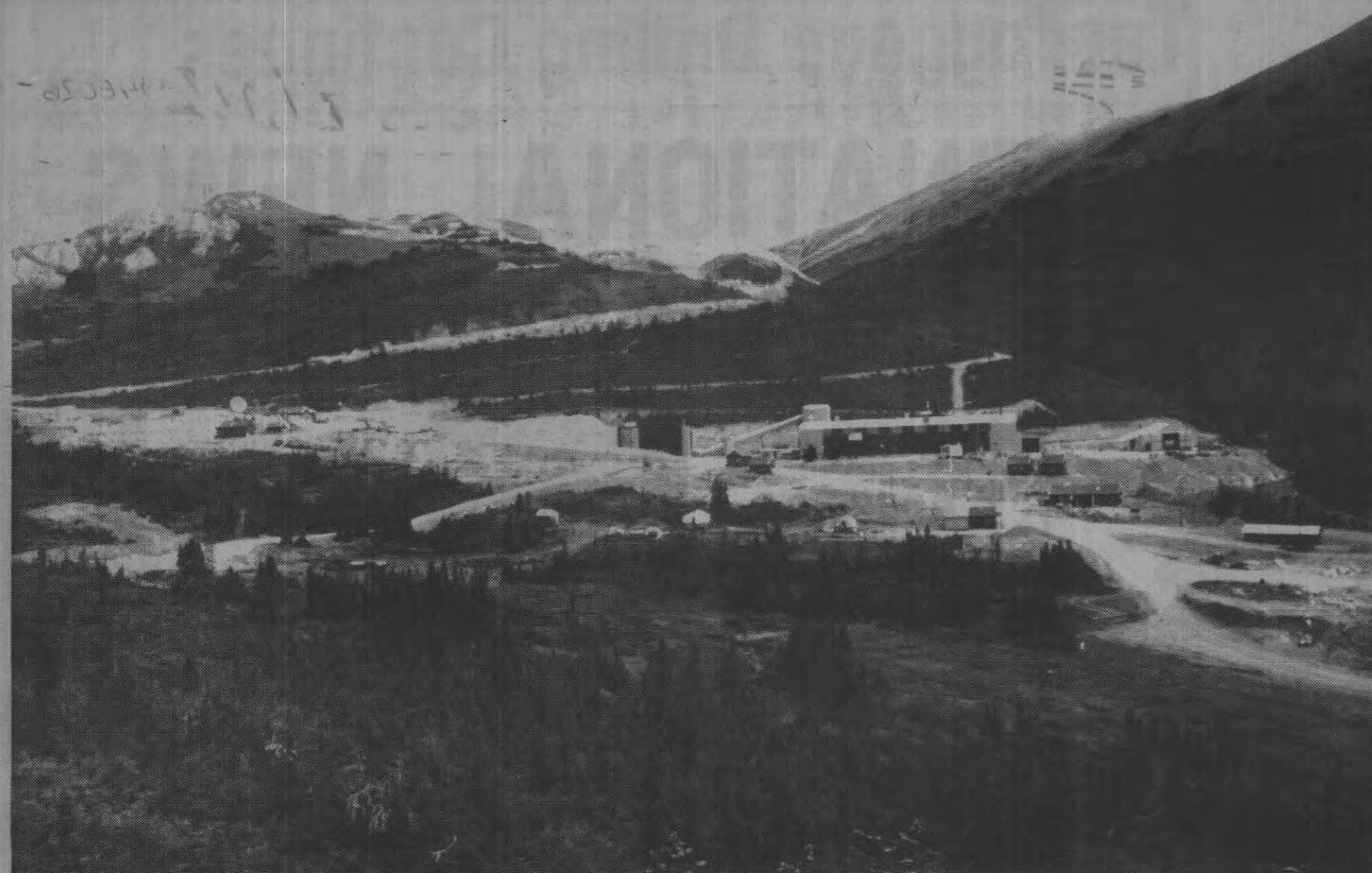
The Baker Mine complex at Toodogone is a fully equipped mining operation complete with 100-ton per day mill. Multinational Resources has an option on the plant and has considered expanding the capacity to about 150 tons per day to service some of the many mines being developed in the area.
