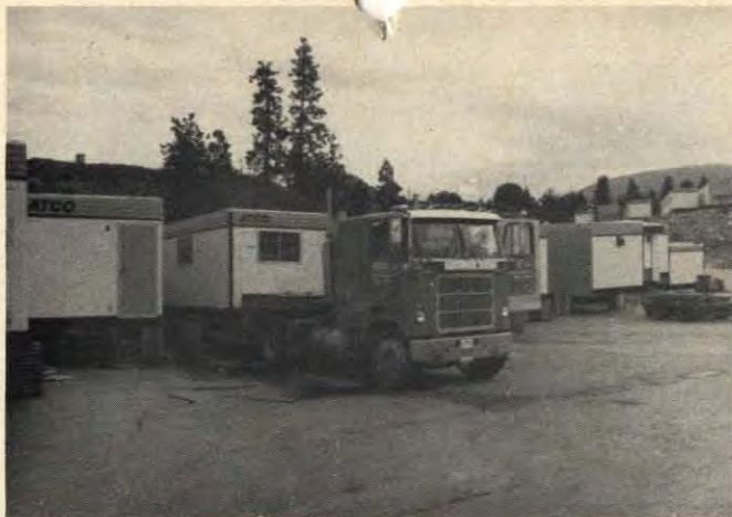
Some of the 27 accommodation units being built at Atco Pacific's Pentiction plant
