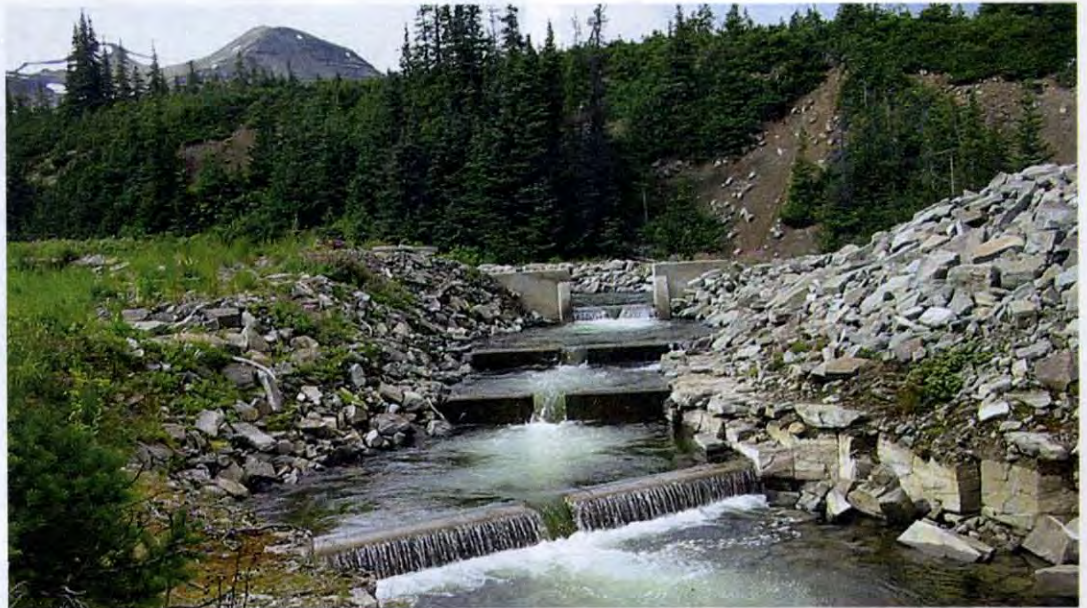
One of three fish ladders built as part of the company’s fish habitat management program, which will be the model for the programs at Kemess North. A new population of Bull trout has been established upstream of the ladders, and the number of Bull trout fry has exceeded the average recorded in the past 10 years.
