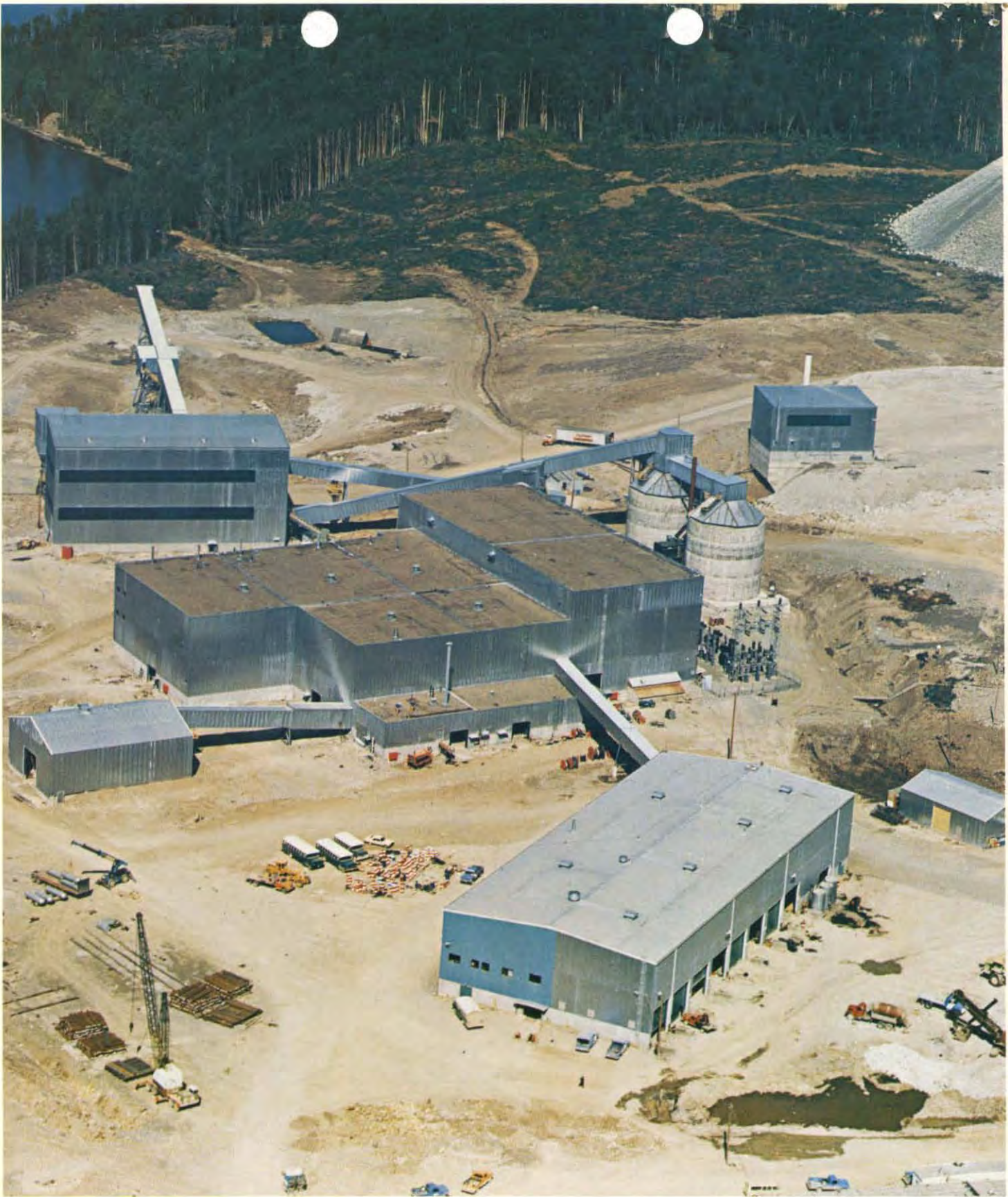
BELL COPPER 1972 Noranda Mines Limited 10,000 T.P.D. Copper, Babine Lake, B.C.
