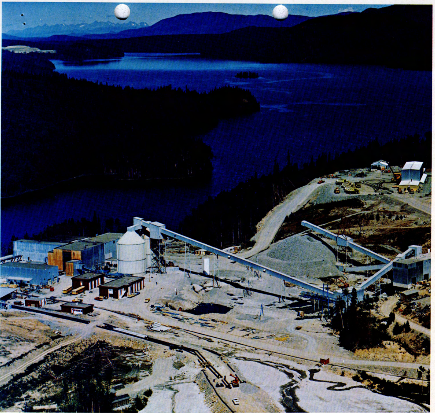
GRANISLE 1972 The Granby Mining Company Limited 14,000 T.P.D. Copper Topley, B.C.
