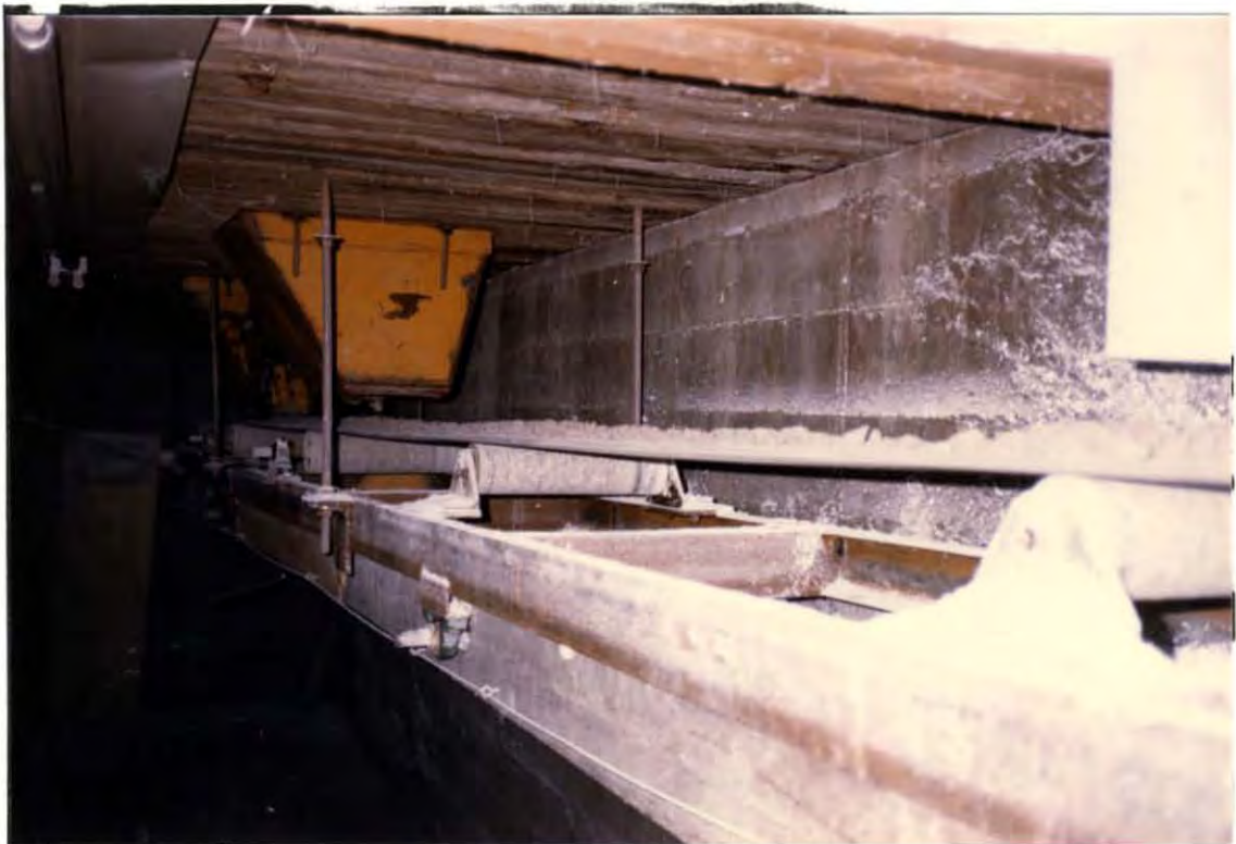
86-Roll 4 - 1 Crushed mill feed entering on conveyor belt.
