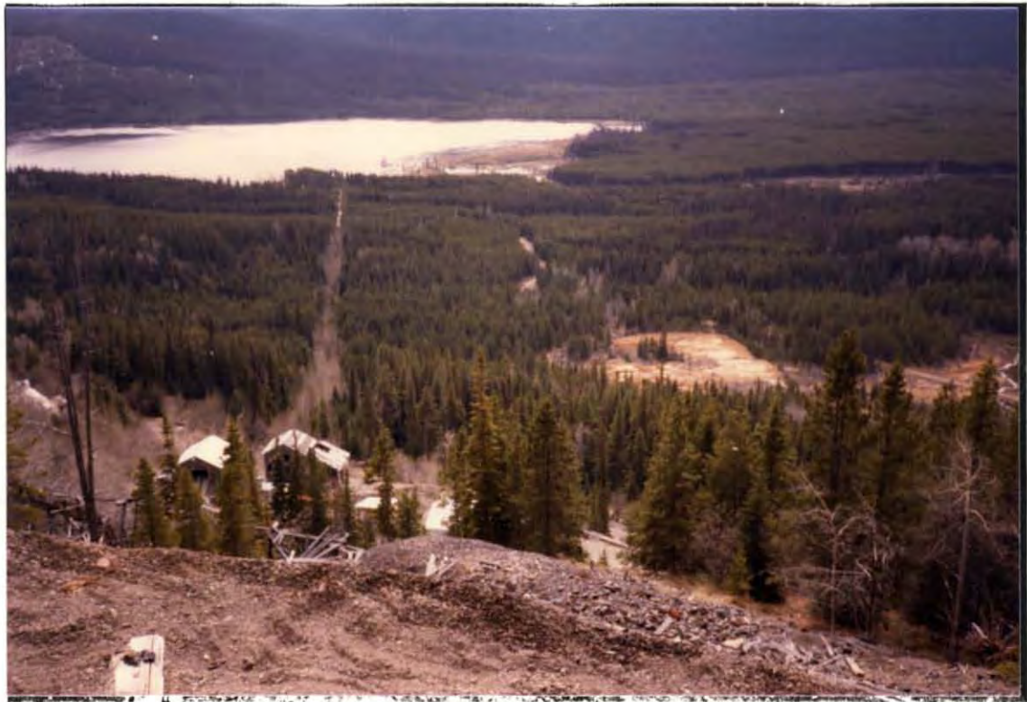
86-Roll 4 - 14 View of the mill, tailings pile and Aldrich Lake. Tailings are alternated with layers of gravel.
