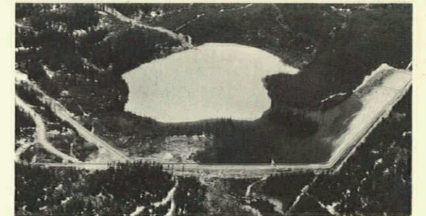
The tailing disposal area showing disposal line on dam at lower side of lake. Floating pumphouse and return water line, upper left side of lake.
