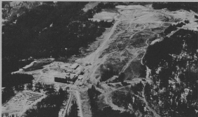
Aerial view of Endako Mines: plant site, center; open pit, upper center; tailing line and main access road, lower center
