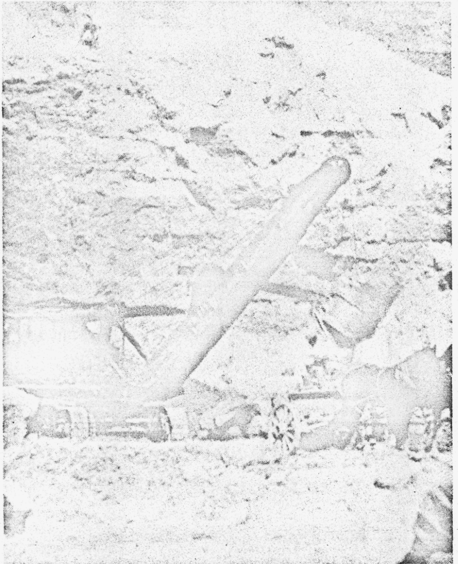
This mechanized shovel was used to dig through 60 feet of overburden to the blue clay. Below that depth each scoop of blue clay yielded gold—until an underground spring broke through and flooded the huge pit. By the following morning, the mine was a lake.
