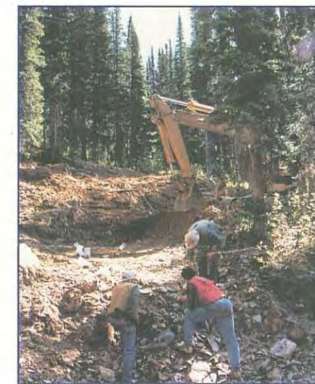
Trenching at Cariboo-Hudson
