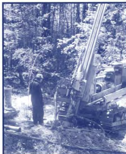
Mineral exploration drilling on Rock Creek Gold Trend Joint Venture project lands.
