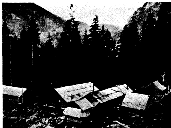
A portion of the Central Zeballos camp. The power-house, new cook-house, and terminal of the aerial tramway are not shown in the picture.
