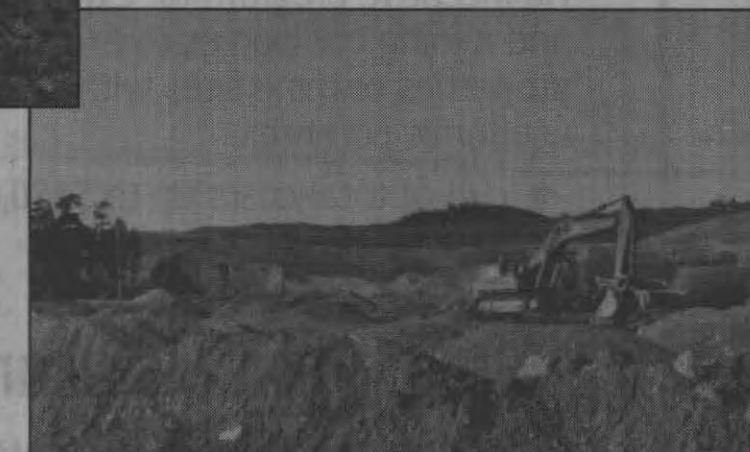
Backhoe spreads stockpiled glacial tills prior to reseeding.
