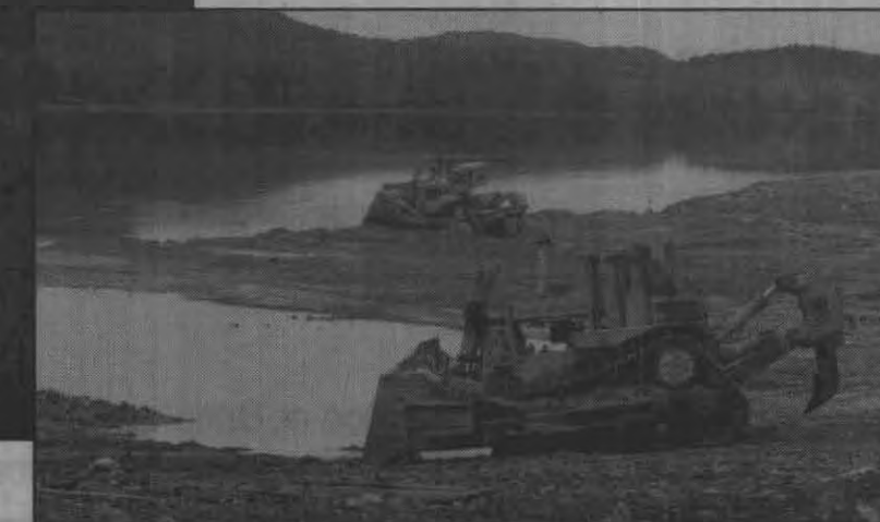
The mine's operating equipment is used to construct bays along the beach dump which create an improved habitat for marine organisms and fish.
