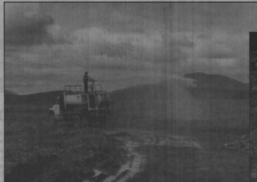
Hydroseeder sprays a mixture of grass seed, fertilizer and mulch on recontoured land.
