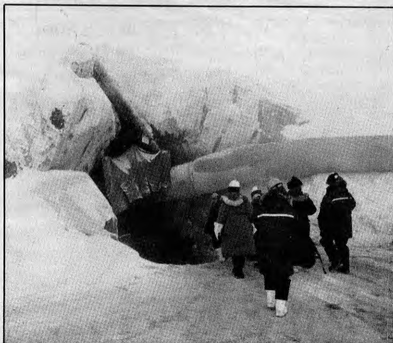
Visitors to the NWT Diamonds project enter the portal of a 1,500-metre tunnel giving access to a diamond-bearing kimberlite pipe located 250 metres below Fox Lake in the Lac de Gras area. Photo, Northern News Services
