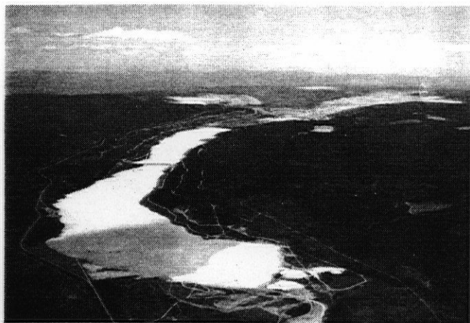
FIGURE 1. Highland Valley tailings impoundment (L-L Dam in the foreground).
