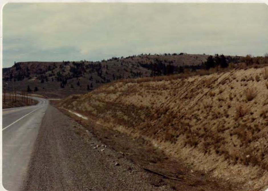
Figure 9B: Relocated Trans-Canada Highway cut seeding. South facing slope. (April, 1980)
