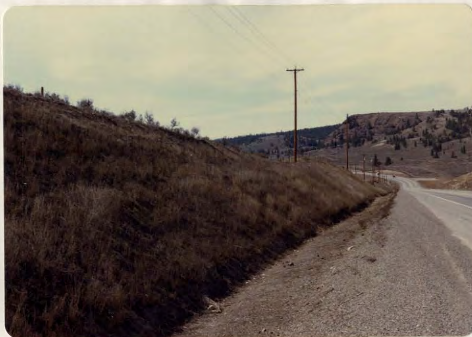
Figure 9A: Relocated Trans-Canada Highway cut seeding. North facing slope. (April, 1980)
