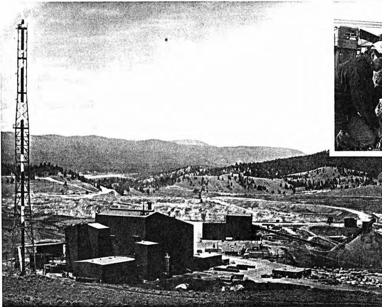
The Afton plant, with the smelter in the left foreground and the concentrator building on the right, and inset examination of ore at the new Ajax open pit.
