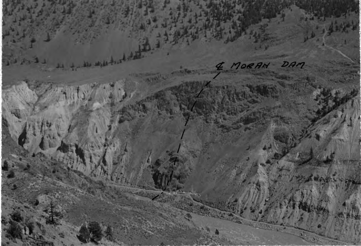
Plate IV A.--East abutment at Moran damsite - with old drilling camp in centre foreground.
