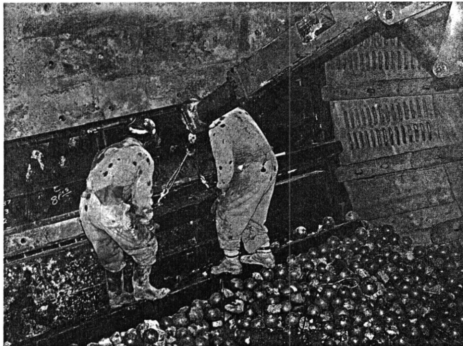
Replacement of SAG mill liners
