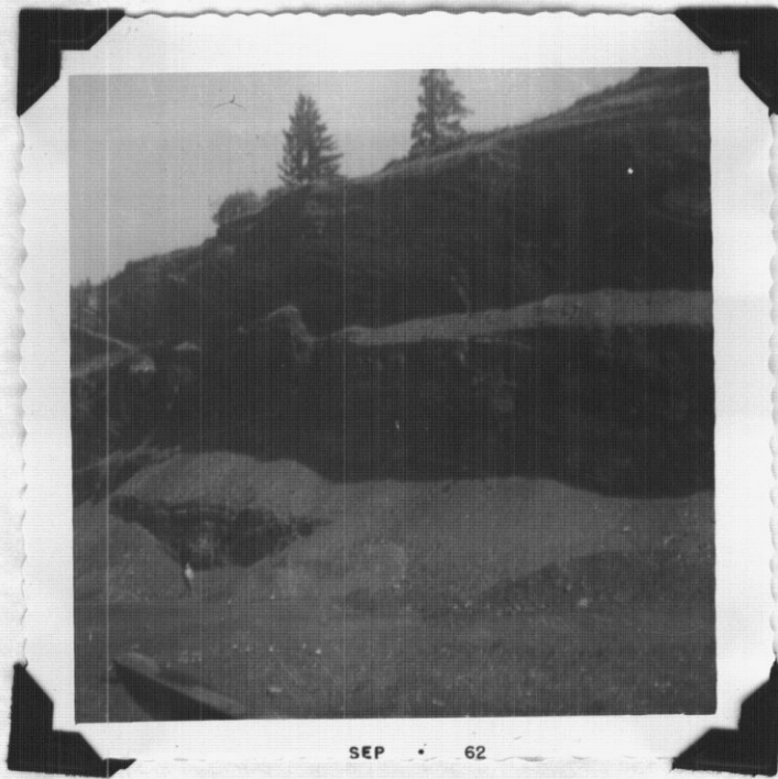
Mullin Pit Coal Measure. Note broken coal on old benches and man standing at toe of exposure.
