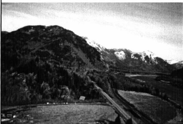
Ruby Creek, BC, Infrastructure Corridor
