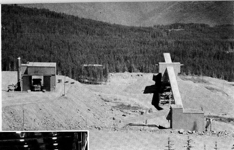
Primary Crusher (left) Primary Screening (lower right)
