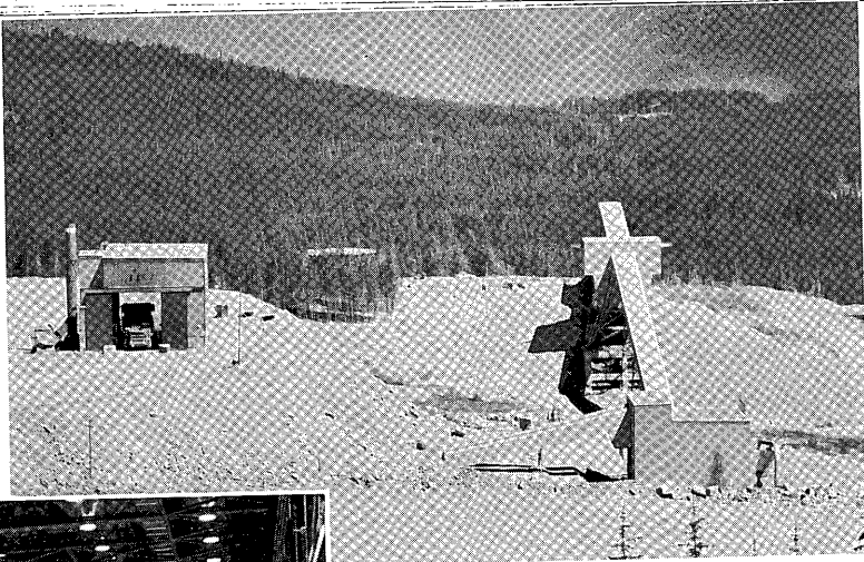
Primary Crusher (left) Primary Screening (lower right)
