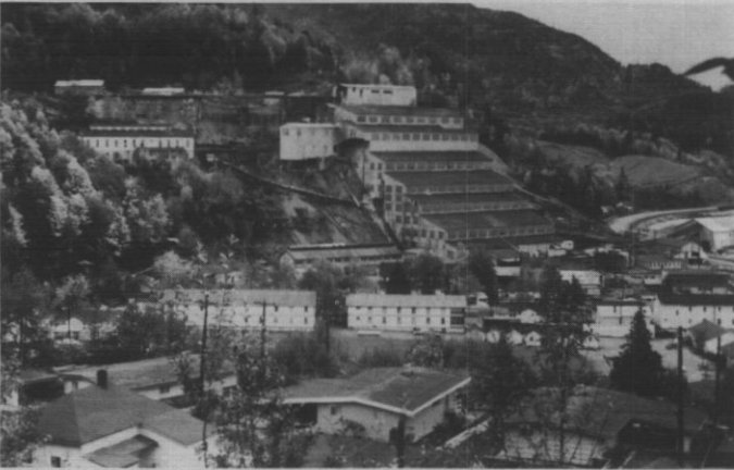
General view South, over upper townsite. Concentrator and Powerhouse in middle distance
