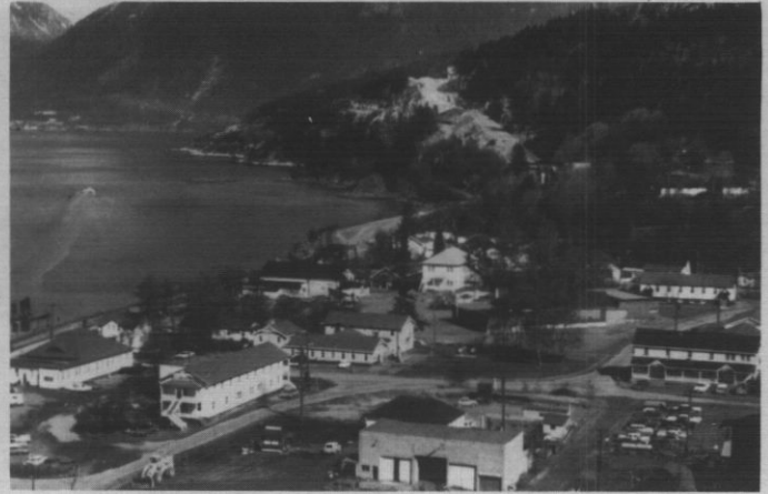
General view North, administration and community buildings in the foreground
