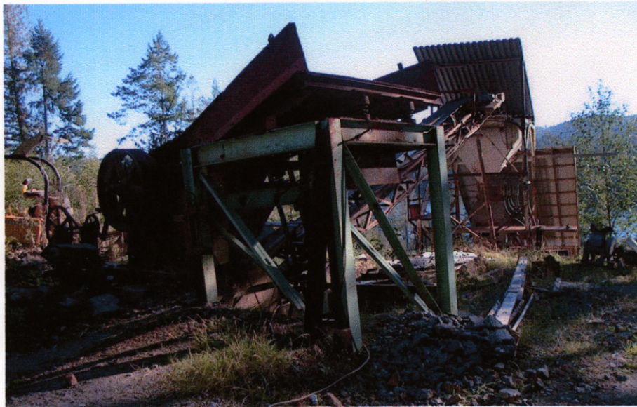
October 3, 2001 - Bob Duker's backyard pilot mill at Texada Island - hopper area
