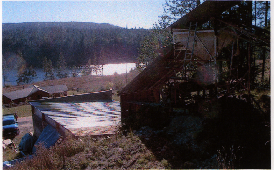
October 3, 2001 - Bob Duker's backyard pilot mill at Texada Island - hopper area
