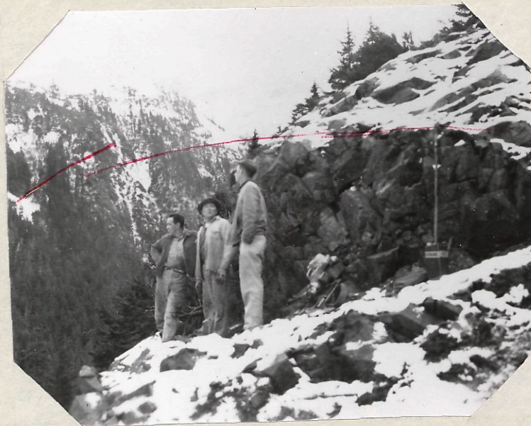
Photo #2 Looking Southerly at cut in Mineralized Basaltic Volcanics. Chalcopyrite occurs along numerous joints. Note Cobra Drill.
