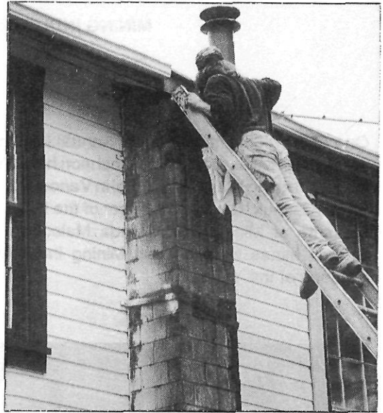
EAVE TROUGH REPAIR ON THE GEO-CHEMBUILDING
