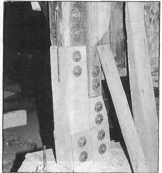
BUILDING AND CRANE-WAY STRUCTURAL POST SPLICES IN THE MACHINE SHOP
