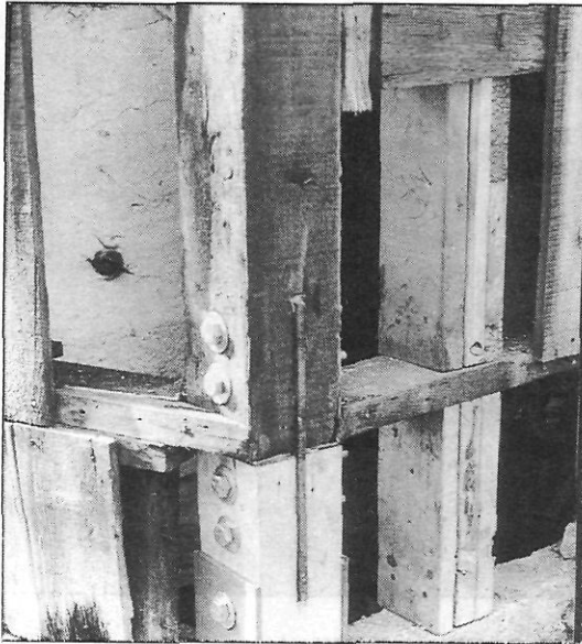
CENTER KERF PLATE POST SPLICE IN MACHINE SHOP
