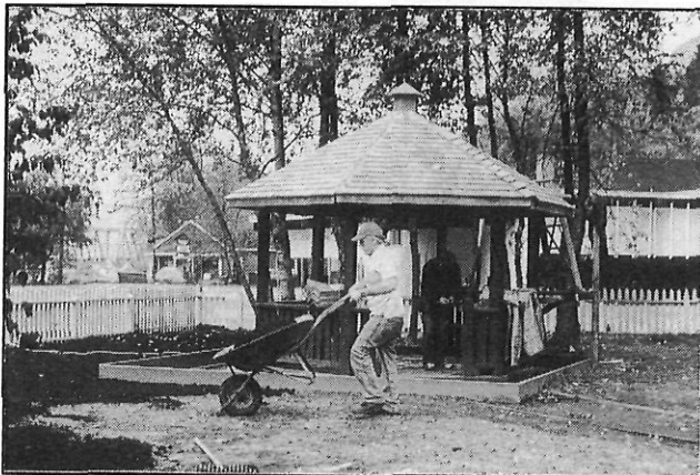
GAZEBO STRUCTURAL AND ROOFING REPAIR AND PARK REHABILITATION IN PROCESS
