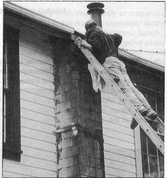
EAVE TROUGH REPAIR ON THE GEO-CHEM BUILDING
