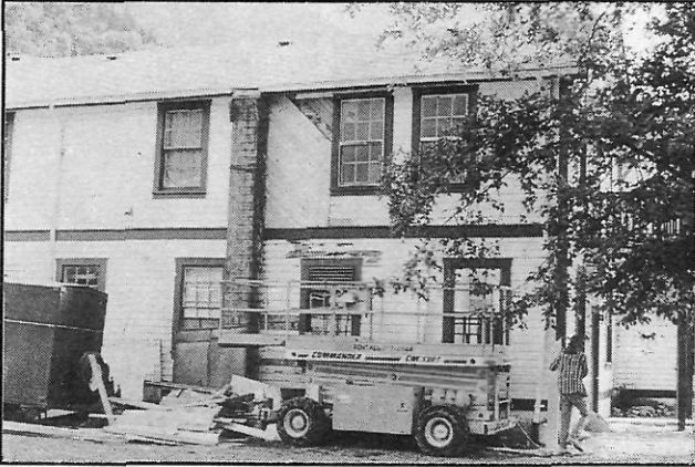
CLADDING AND SHEATHING REPAIR PRIOR TO PAINTING THE GEO-CHEM (COOKHOUSE)
