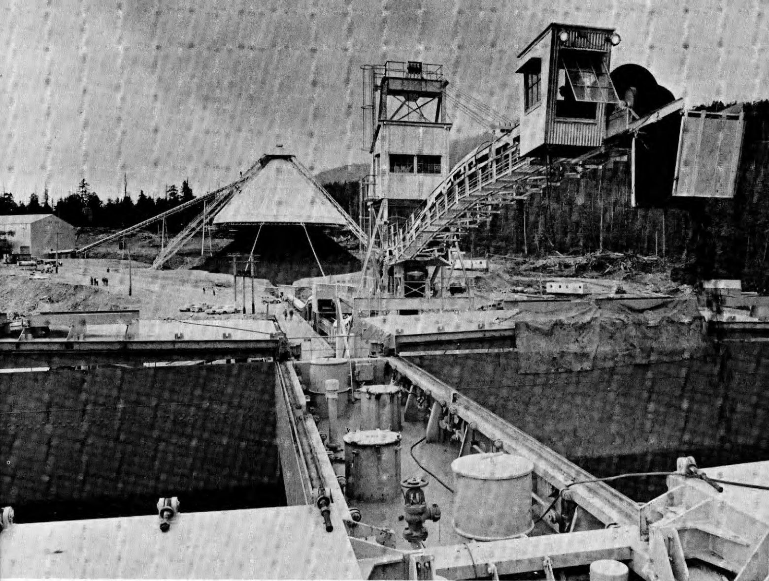
Loading the "Yawatasan Maru" at Toquart Bay. Steel for the conical cover of the live concentrate stockpile was provided along with several other major construction units by the Western Bridge Division of Canada Iron Foundries Ltd.
