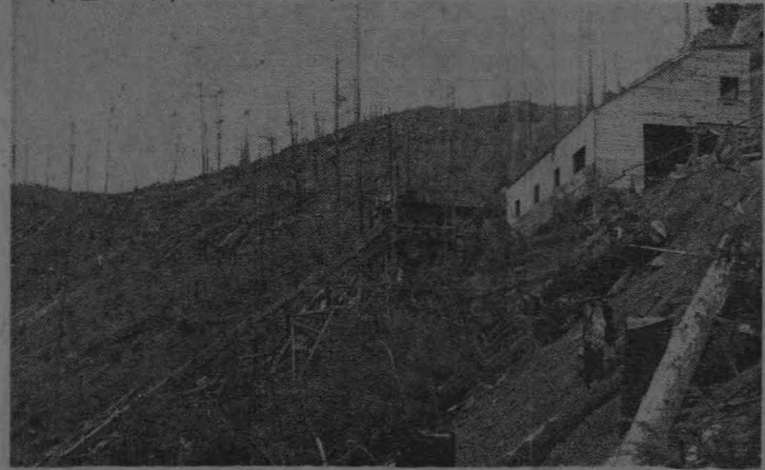
Shops, ore chute at Blue Grouse Mine cling to steep logged hillside.
