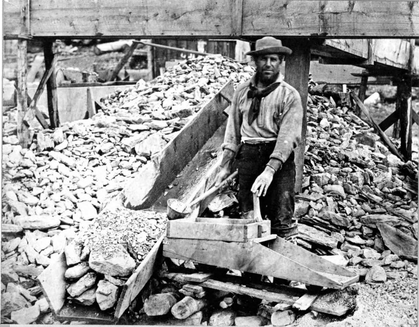
Bill Phinney with a gold mining rocker at Old Caledonia on Williams Creek, ca. 1868. (Catalogue no. 767)
