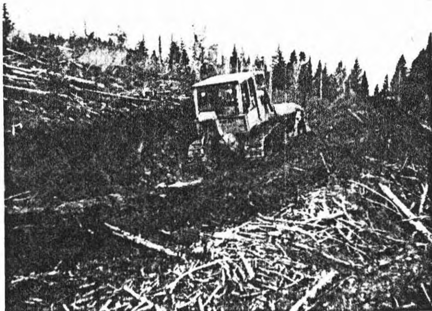
Rea Gold. Ken Vanoyole's D6C bulldozer trenching the Hilton showing, supervised by Roy Nichol and Ralph Shearing, Oct 83
