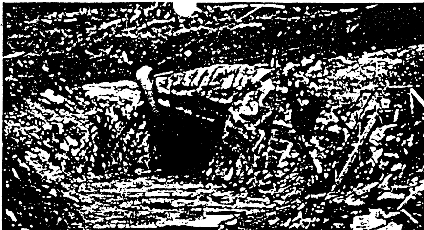
An adit driven during 1976 encountered the mineralized zone 1,300 m into the hillside. Drifts were driven into the mineralized zone, and into the hangingwall, for detailed diamond drilling
