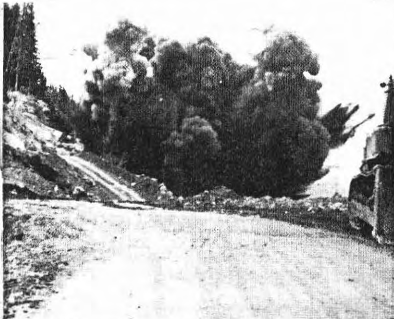
Goldstream. Open pit blast
