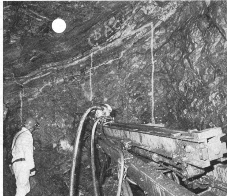
Goldstream. Slope preparation drilling; photo shows slope of back which follows top of ore zone
