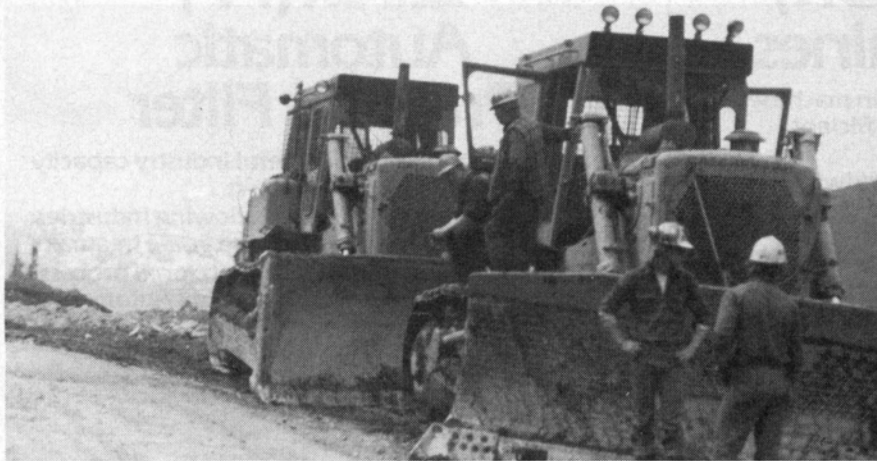
Goldstream. Waiting to blast at the pit
