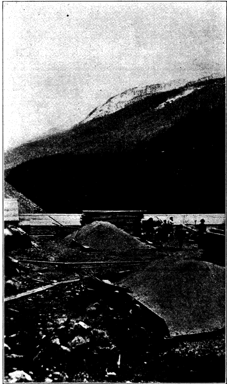
Building Materials on Site of New Concentrator
