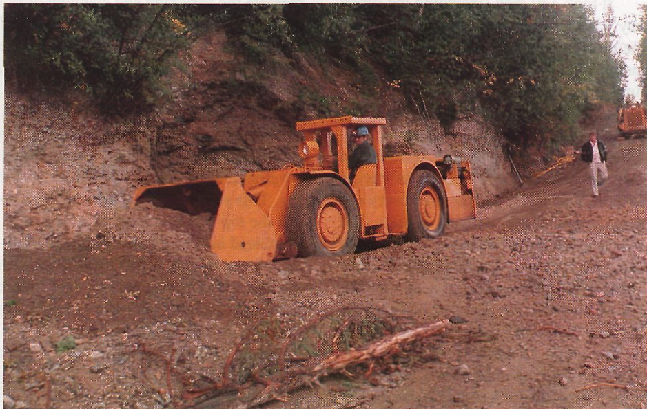
Scoop tram busy at work
