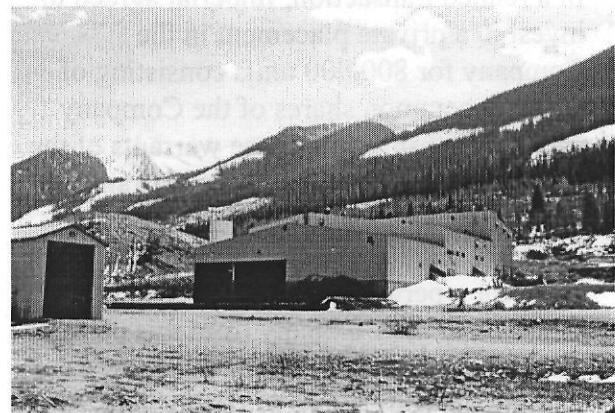
GoldStream 1,000 mtpd Flotation Mill (May 2002)
