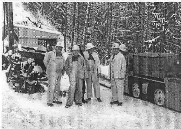
Executives from the Joint Venture Visit the 1025 Level Adit Drive at Willa (circa 1985)
