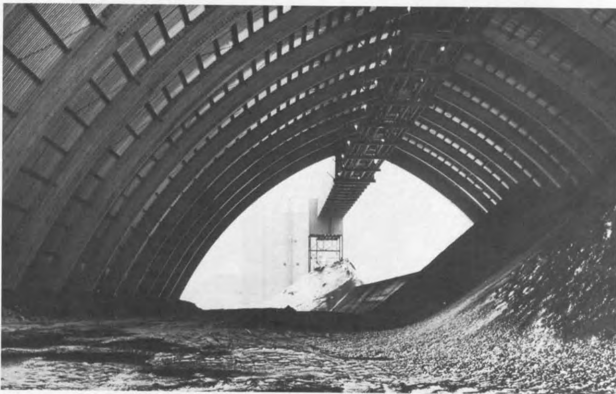
At Fording, product coal is loaded out onto unit trains from this storage building.
