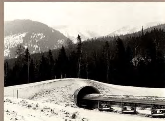
Innovative Line Creek conveyor design permits safe crossing by wildlife.
