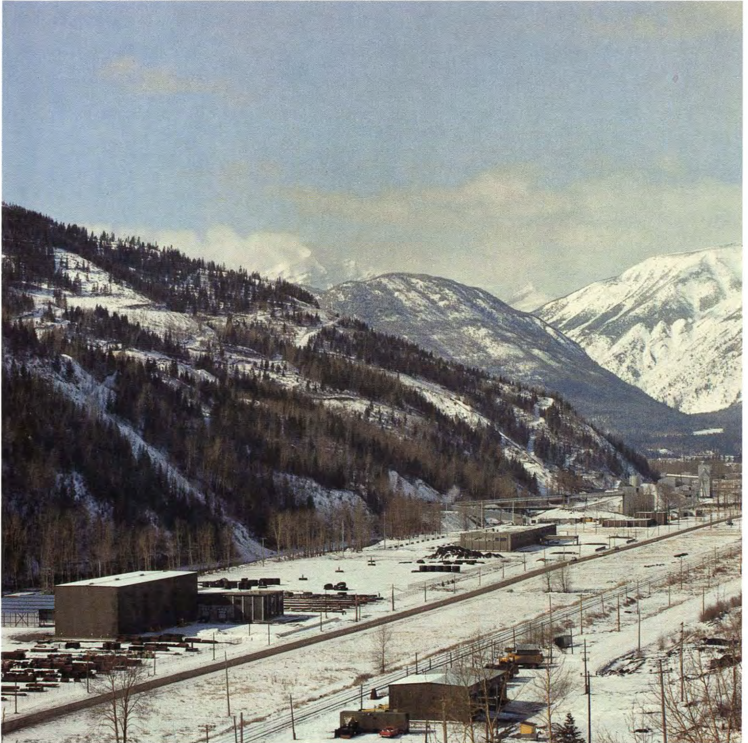
New warehouse and administration building form part of a fresh image for the Michel Valley at Sparwood.
