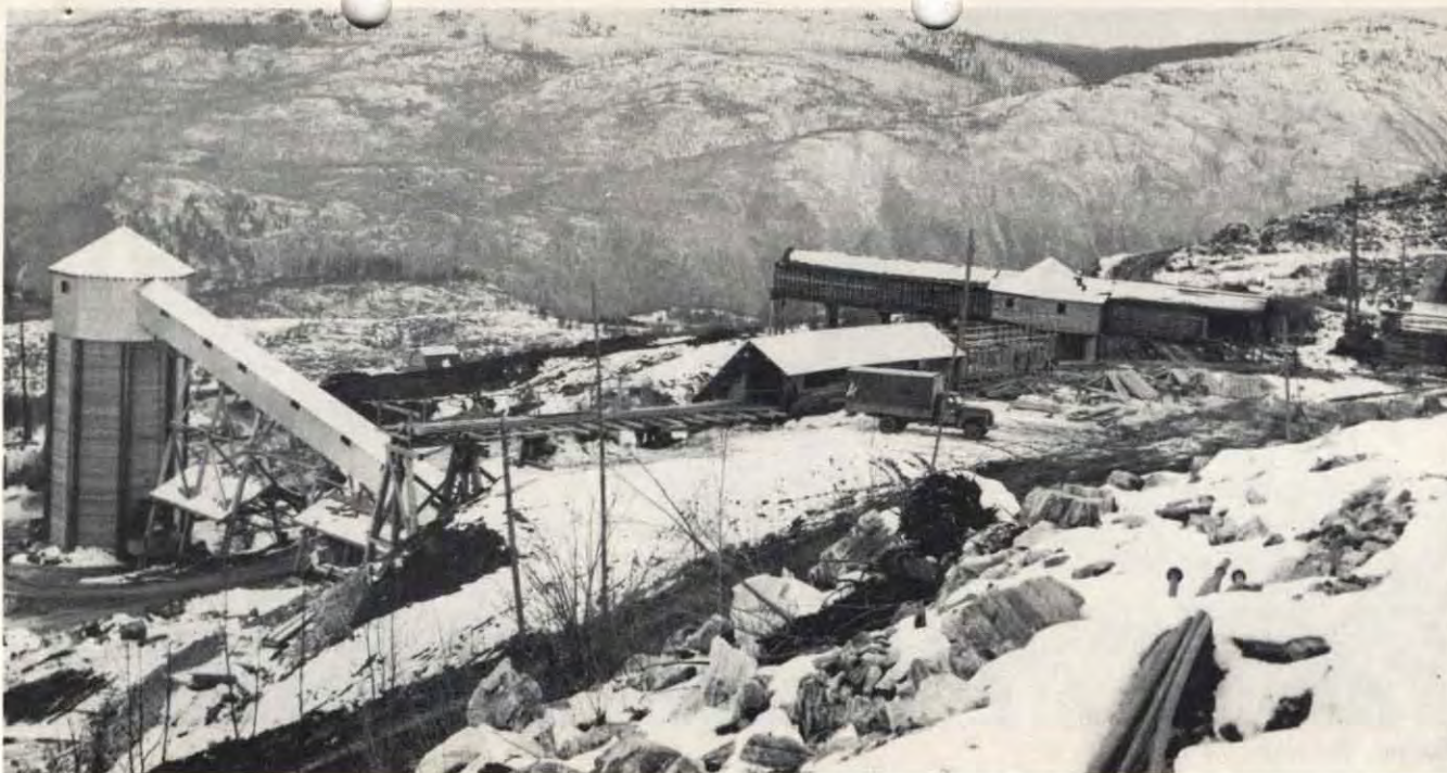
Salmo: Jersey lead-zinc mine portal area
