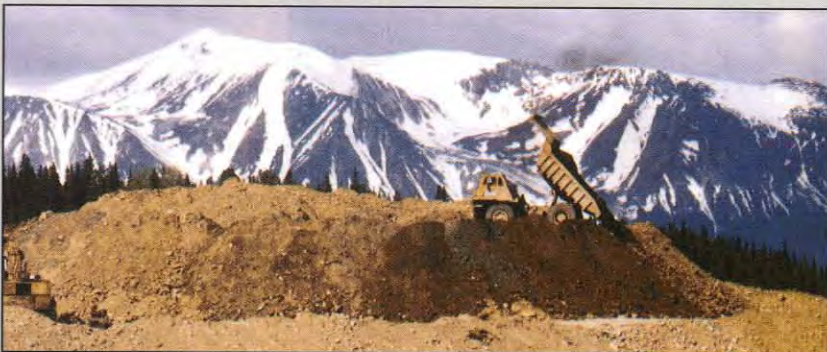
This 50,000 cubic yard ore stockpile at Pine Creek was mined and processed in 1987.
