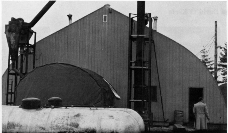
Rear of Aurun's pilot plant showing converter furnace
