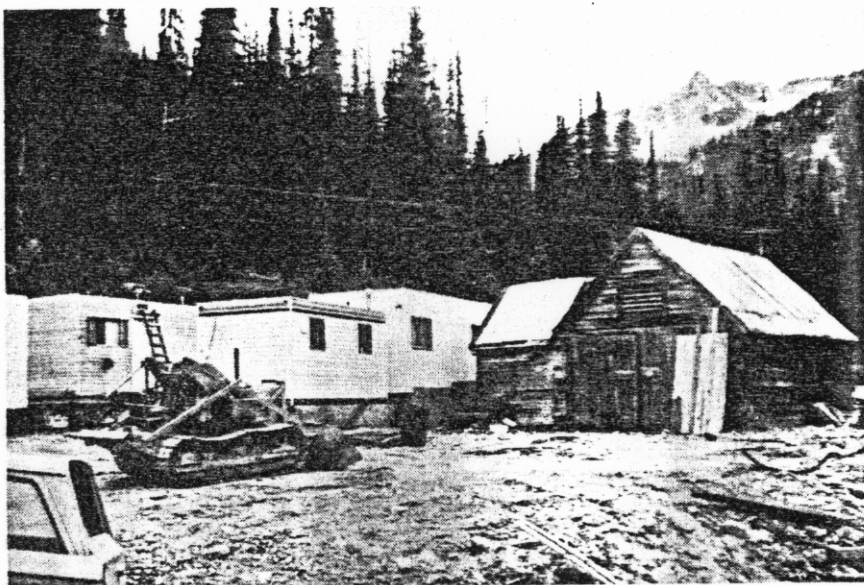
New trailer units in sharp contrast with picturesque old machine shop as finishing touches ready David Minerals camp for company's Kokanee Glacier Park Mine.
