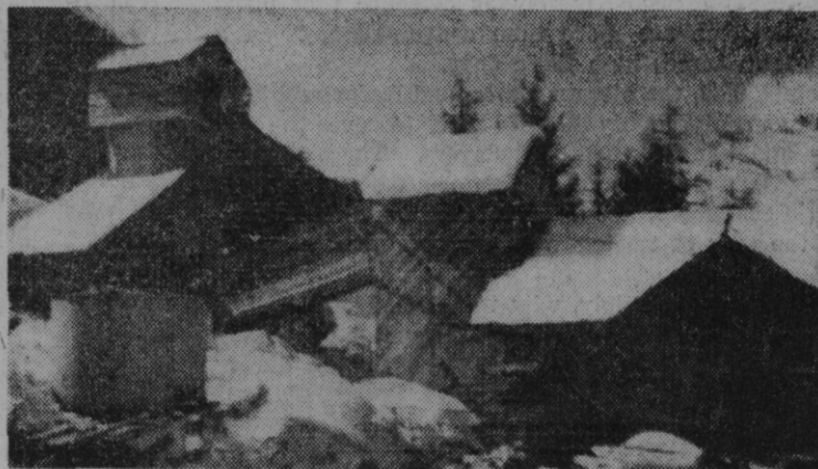
Crusher and Power Houses
