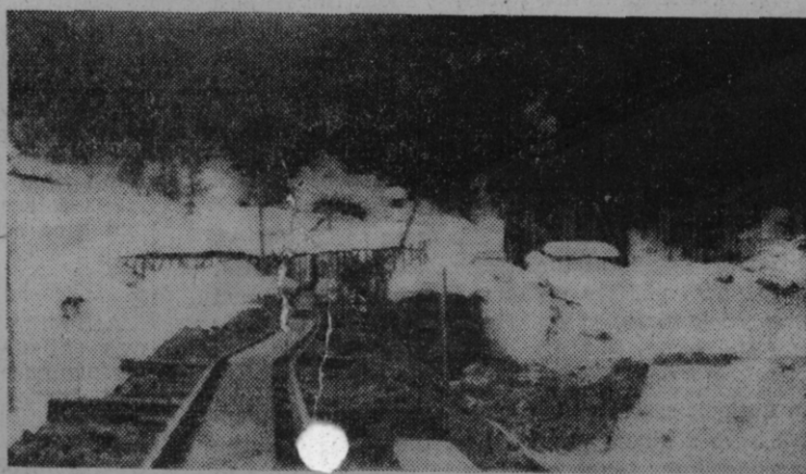
View Towards Mine Portal
