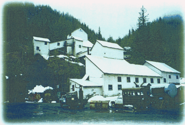
100%-owned, 100 TPD, Full Flotation Mill at Sandon, BC
