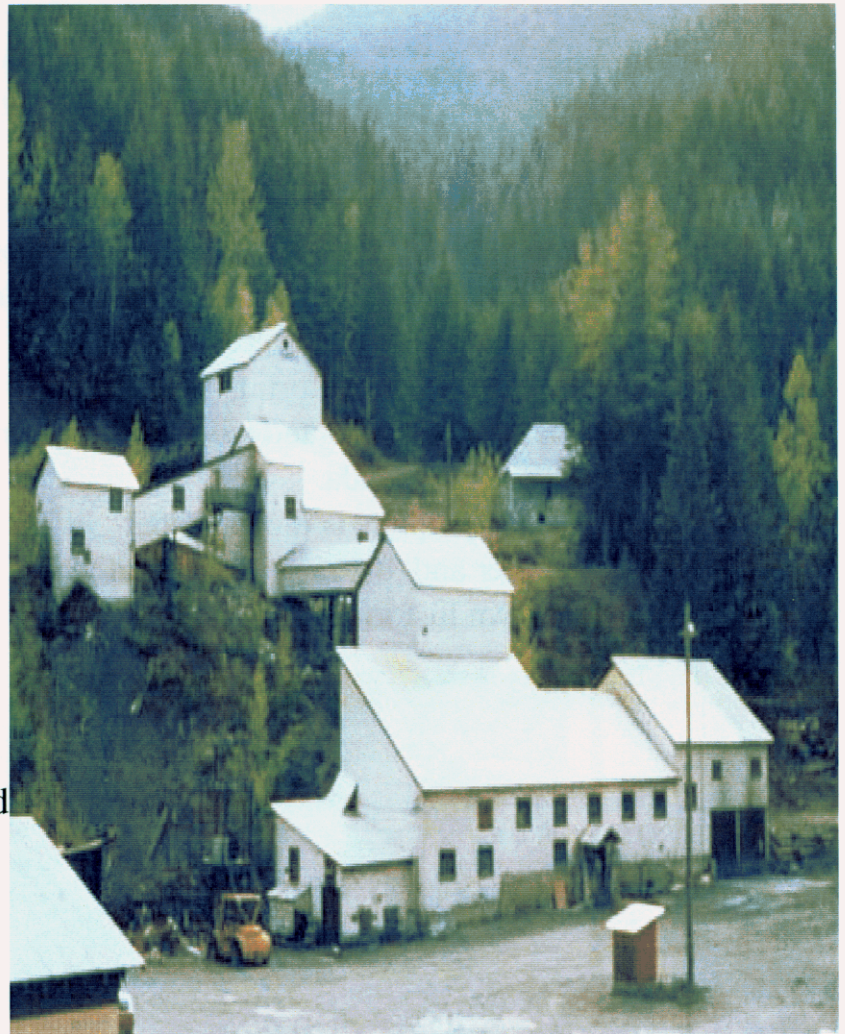
The 100 ton per day Klondike Gold Mill at Sandon in the Slocan Mining Camp
