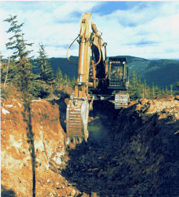
Trenching the Thea Gold property, Purcell Mountains.
