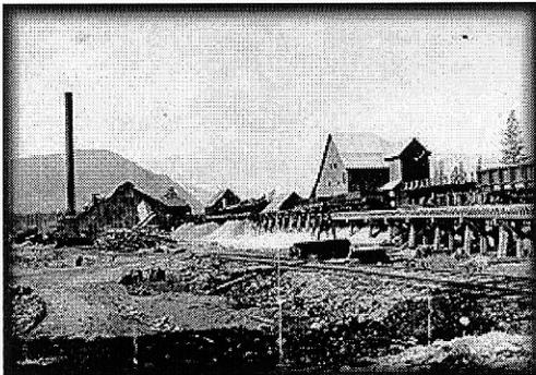
In 1903, work began on a small smelter at Marysville five miles (8 km) from Kimberley. The smelter was "blown in" early in 1905. Initially a small profit was made but the process did not solve the problems encountered with the Kimberley ores. The difficulties in smelting the Kimberley ores continued because of their zinc content and the smelter closed permanently and the mine was shut down for a short time pending financial restructuring.
