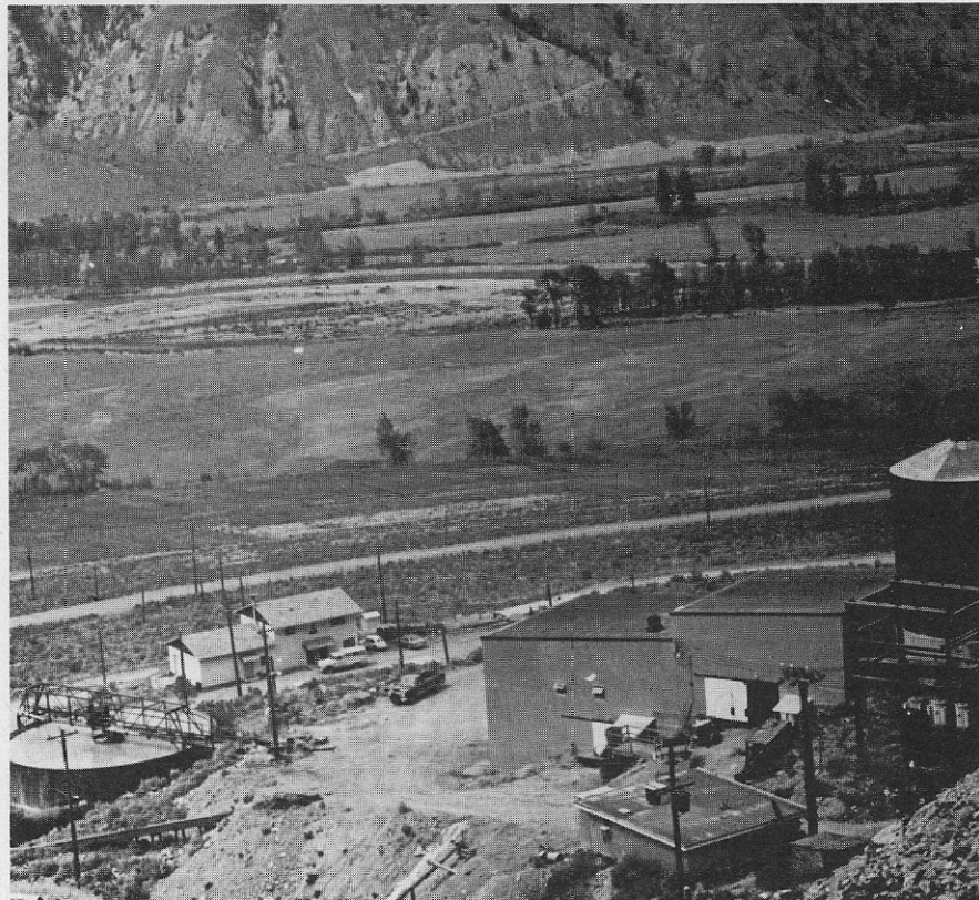
DANKOE: Mill (right) and offices buildings at the mine overlook the Similkameen River Valley. The mill is about 4400ft from the main haulage way at the 2200ft level.
