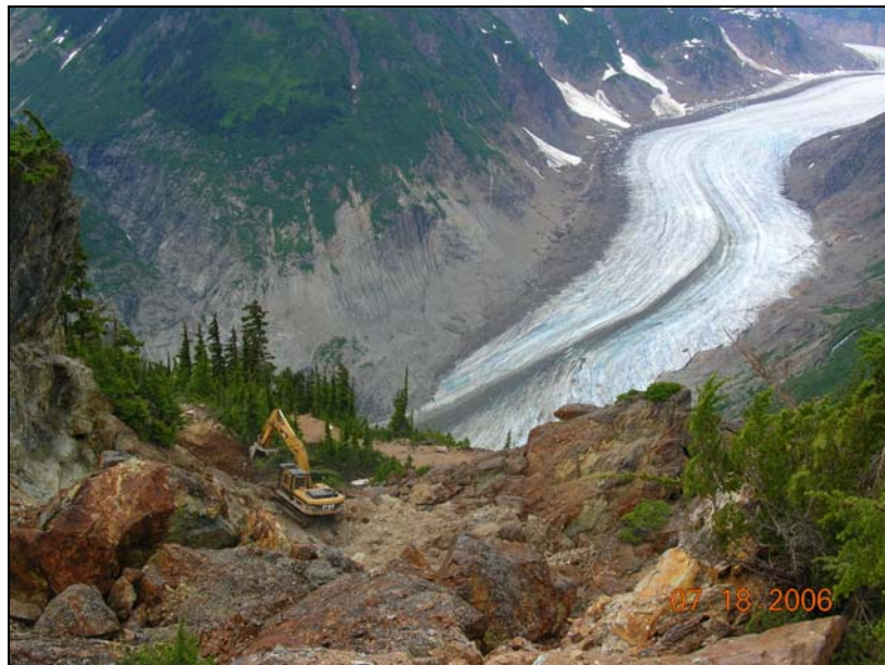
Figure 7.3 – Drill Pad Preparation on a Steep Hillside above Salmon Glacier
